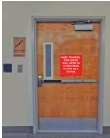
Current delayed egress signage
